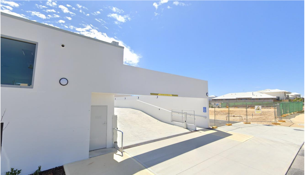
Previously installed bulkhead with 2.3m clearance – source: Google Street View
